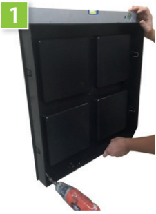
▪ Attach back frame to wall
