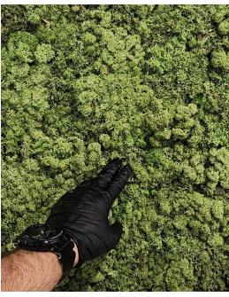
If the provided measurements were incorrect, you might have too much material to fit the wall. If that's the case, you will need to measure and cut away any extra material for your panels to fit properly. This can be done by measuring and marking a line with a straight edge and then carefully using a box cutter / sharp blade to cut along the back side of the panel and through the moss.
